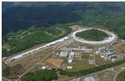
Photo 1. SPring-8 synchrotron radiation facility (circular accelerator surrounding a small mountain) and SACLA X-ray free electron laser facility (linear accelerator).
